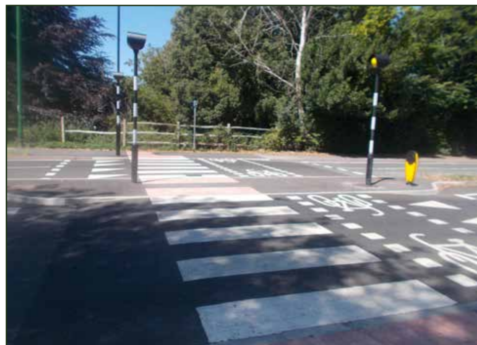
What can be done! A new Zebra crossing on Avenue de Chartres close to Chichester College. Note the cycle route
