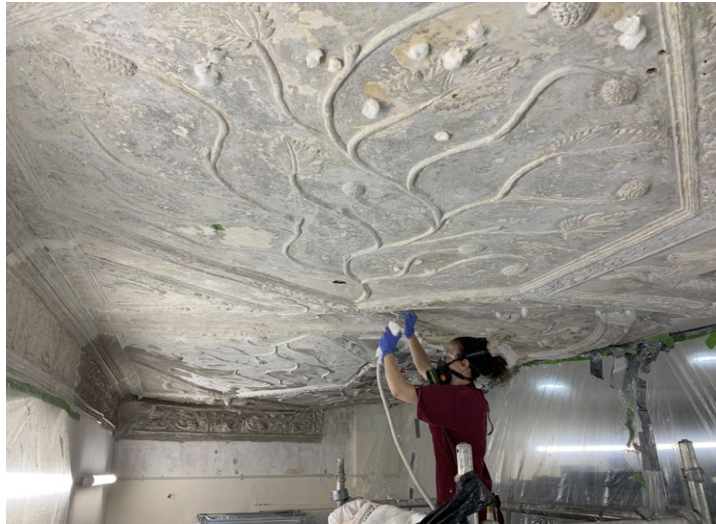
Conservator Jenna Burrell uses a steam cleaner to remove layers of paint.
