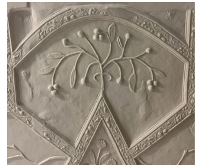
One of the panels in the main room after treatment.
