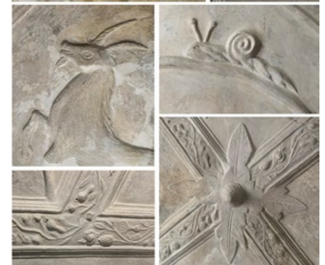
Close up of different details revealed after paint removal.
