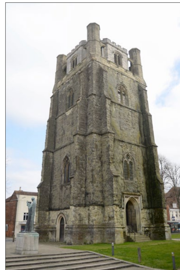
Chichester Cathedral has the only medieval Bell Tower in England. It dates from around 1400, is 107 feet high with 8 feet thick walls.
